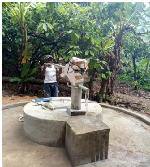
Testing the pump in Than Town
