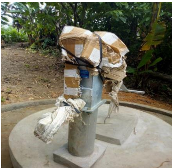
Completed Afridev hand dug well in than town
