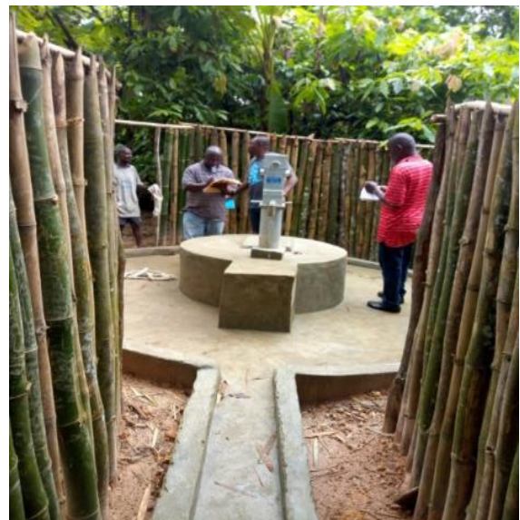
Verification of completed well in Than Town.
